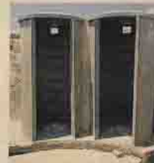
Pre-fabricated low-cost community toilets.
