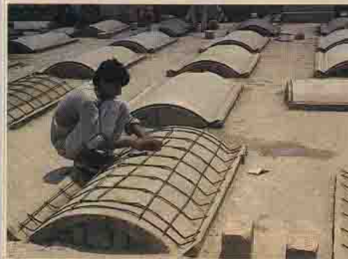
Making ferrocement panels for the toilets.
