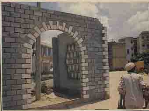
An archway made of concrete filler blocks.
