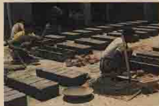
At the Nizamuddin centre, making concrete filler blocks for use in low-cost housing.
